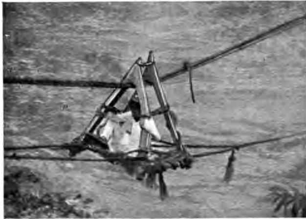
CRADLE ON ROPE BRIDGE
